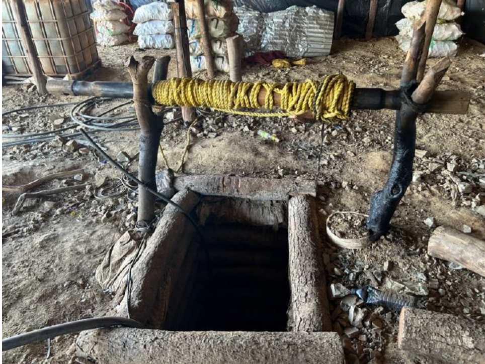
Photo 16: Cameo Main Shaft: Deeper underground workings use wood cribbing to secure the shaft and a simple rope crank to remove material.
